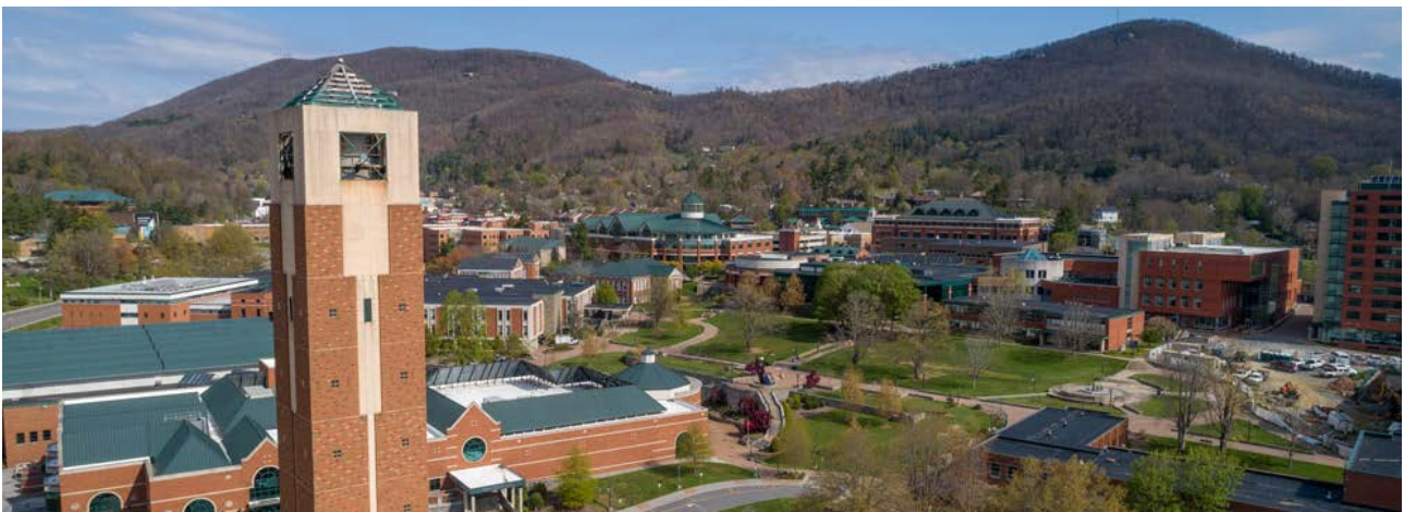
The university's steam plant provides both heating and hot water for much of campus through an approximately three-mile steam loop. The majority of App State's heating requirements are provided through the production of steam via the plant's four boilers.
