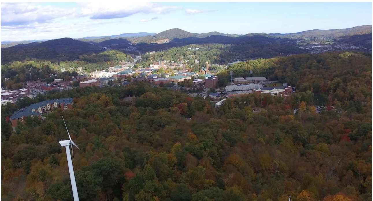
The 100 kW Broyhill turbine was the largest wind turbine in the state of North Carolina when it was installed on campus in 2009. Ten years later, it reached the milestone of 1 million kWh of emissions-free energy.
