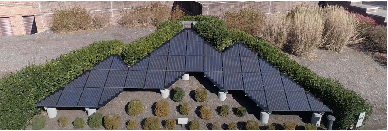
The shape of the photovoltaic array in front of Peacock Hall reflects our location in the Blue Ridge and our Mountaineer spirit. At 3,333 feet above sea level, App State is the highest elevation of any university east of the Mississippi River.
