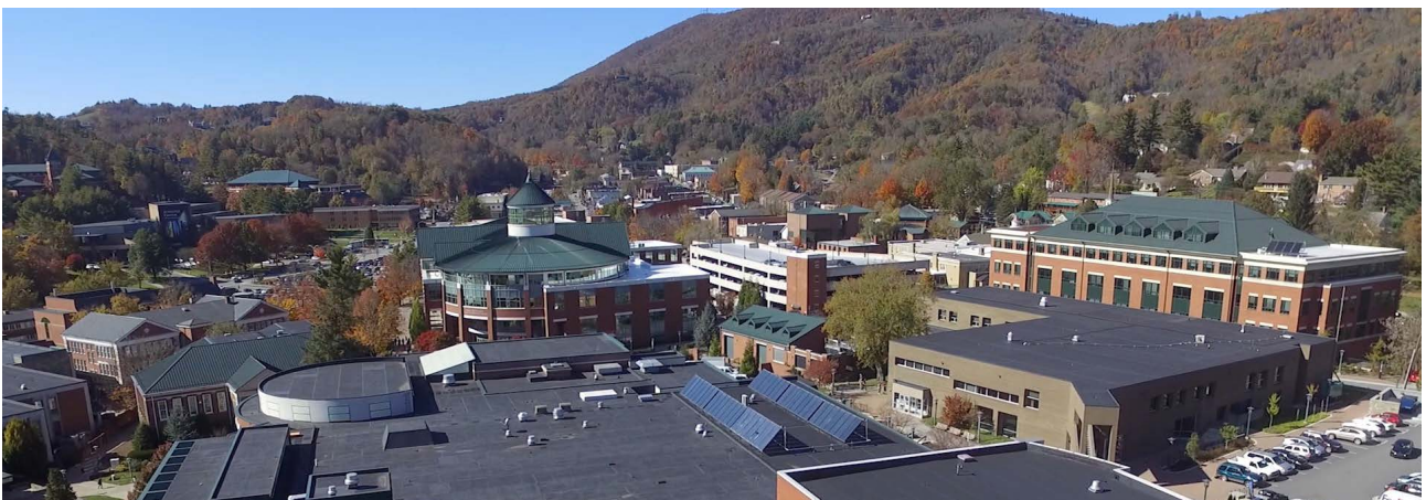
The 35-panel Plemmons Student Union solar-thermal system, pictured in foreground, was the first large-scale system installed on campus in 2009. This system preheats water used in restrooms, fitness center locker rooms and the building's food service areas. The most recent solar-thermal system installed on campus, pictured on the right, is located on the Reich College of Education (RCOE). This system uses four panels for preheating water for RCOE restrooms.
