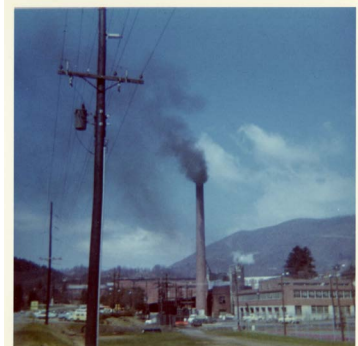
The original campus steam plant smokestack was demolished in 1973.
